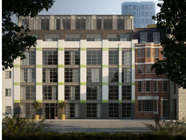
The Askew Building and Abernethy House
