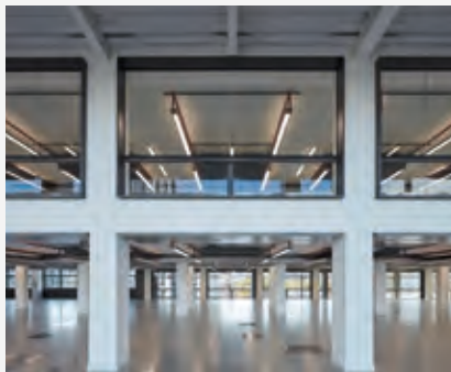
AUG 2018 Phase 2 achieves practical completion
