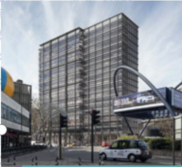
10 The Bower Old Street EC1 Office and retail refurb and extension
