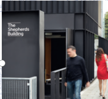
4 Shepherds Building W14 151,000 sq ft office building
