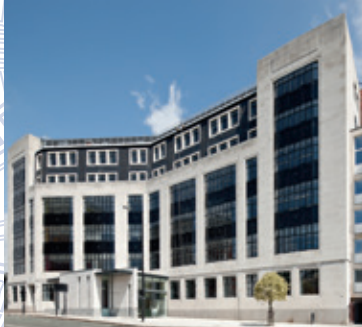
5 Enterprise House W2 45,000 sq ft office building let to Network Rail
