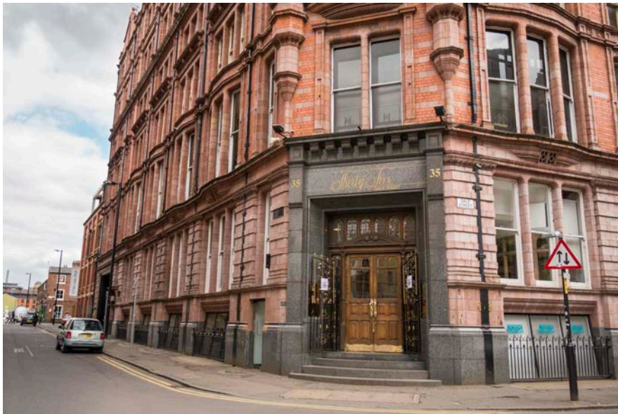
Dale House, Manchester
